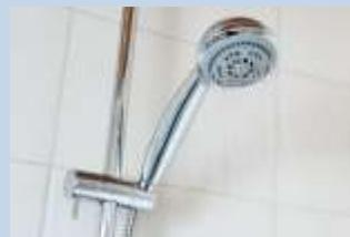
Faucet heads are prone to getting clogged with buildup and can lead to low water pressure. Remember to clean faucet heads often to maintain proper water flow. Most faucet heads are hand tight and can be easily unscrewed by using your hand. Clean thoroughly then re-install the faucet head just hand tight. If needed, use pliers to tighten a little more but remember to use a rag to protect the faucet head from scrapes.
